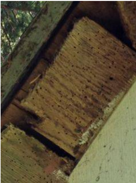
Photo 34-1 Insect holes in wood.
