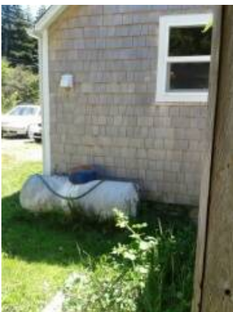
Photo 24-1 Propane tank against house
